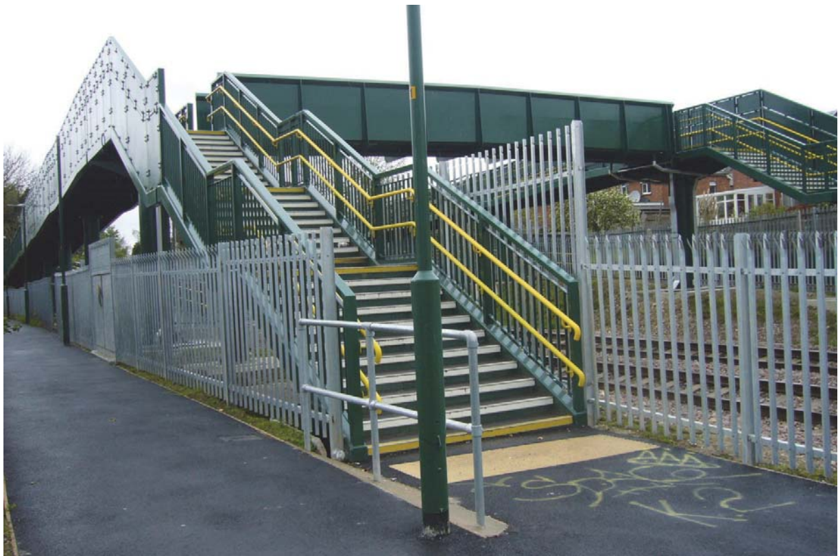
Two views of the new footbridge over the railway at the top of Beards Lane.
